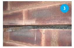
Push helical crack stitching bar into grout, to approximately two thirds of the slot depth. Trowel displaced grout to firmly encapsulate the bar.
