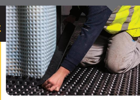
Wykamol Corner Tape is a 150 mm wide tape with many uses, but most commonly used to seal membranes from walls to floors and fixing perimeter drainage channels in place.
