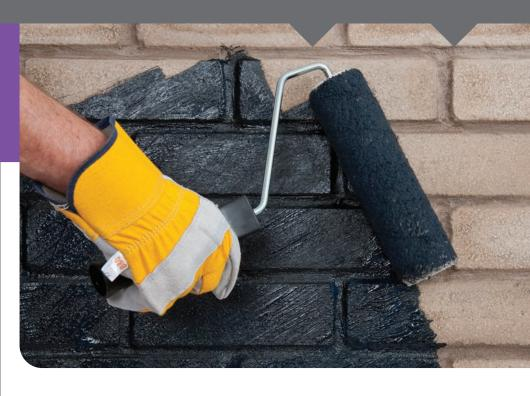
Technoseal acts as a barrier against vapour, damp and water. It is safe to use in portable water and can be applied to pond lining as a waterproof barrier.
