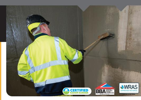
When mixed with clean water and applied correctly, Wykamol Tanking Slurry forms a permanent waterproof coating to the concrete and masonry and is easily applied by brush, roller or spray.
