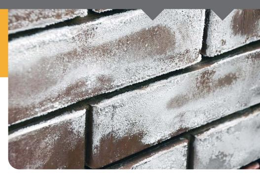
**Salt Neutraliser** is an aqueous solution based on ethanoic acid with an added surfactant. It has been specifically developed to overcome the problem of salts in mineral building surfaces.
