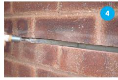
Make good the wall chase to disguise the slot. Repair cracks between the helically reinforced masonry with Crack Sealer Plus.
