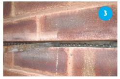
Push helical crack stitching bar into grout, to approximately two thirds of the slot depth. Trowel displaced grout to firmly encapsulate the bar.
