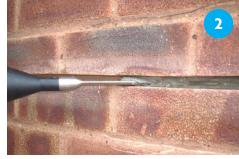
Clear loose debris from slots and flush thoroughly with water and insert bead of WHO 60 grout.
