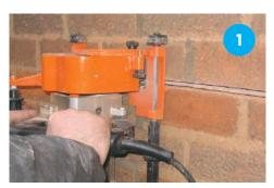
Chase horizontal slots at 300mm intervals that extend 500mm on each side of the crack.
