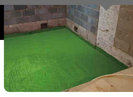
Wykamol Liquid Gas Membrane (LGM) is a single pack, elastomeric liquid rubber membrane, specifically designed for a range of vertical and horizontal construction surfaces, generally as follows. LGM will cure to form a tough, flexible material acting as an effective barrier to the passage of vapour, damp, water, Radon and Methane gas.
