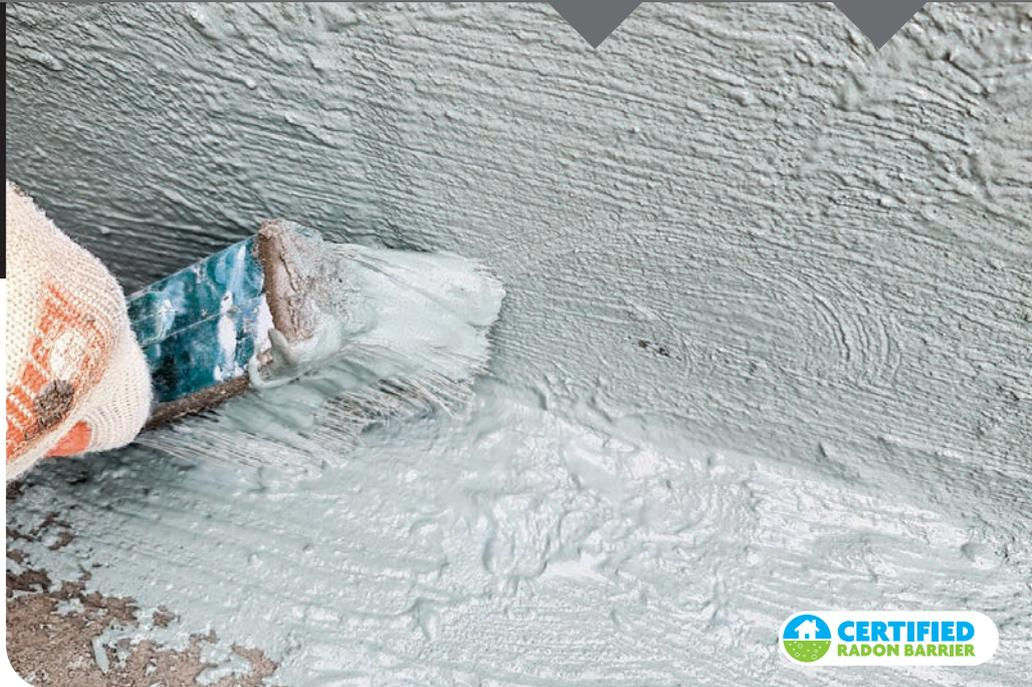
HydraFlex is a two-component flexible coating made of a cementitious powder and a high concentration liquid polymer.
