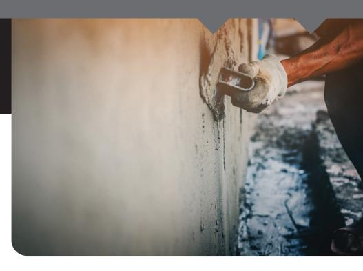
The product cures to produce a high performance, Universal Mortar, multipurpose, fibre reinforced, fair faced levelling coat, render and profiling mortar, with enhanced waterproofing properties.
