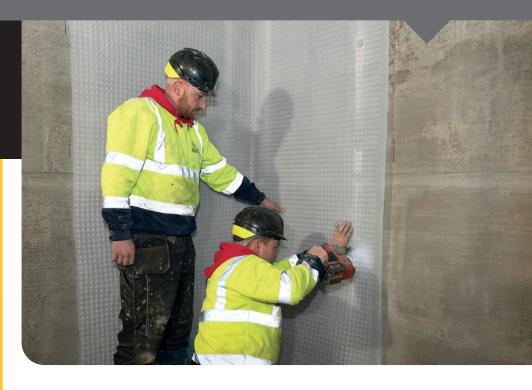
They ensure a water tight application of the Wykamol Cavity Drain Membrane Systems. Wykamol Plaster plugs are of a high quality and can be used in a range of applications and on multiple substrate types. The tailor made Thermoplastic Elastomer seal ensures application of the membrane is water tight.
