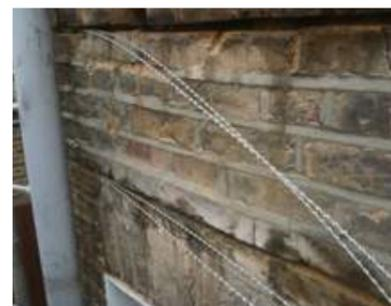
The design principle is based on the formation of a deep beam within the brickwork by the insertion of two chords of reinforcement: the lower tension chord and the upper compression chord (formed by the combination of the grout encased wires and the surrounding masonry). The unreinforced courses between these two chords can be seen as the equivalent to the web of the beam.
