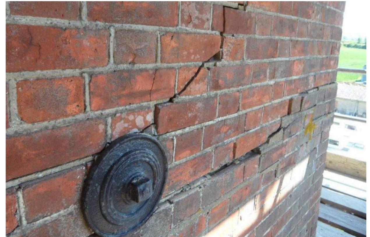
This technique generates an in situ reinforced, deep masonry beam. In order for the reinforced beam zone to accommodate the imposed flexural forces, it is necessary to repoint loose mortar joints and to deep-resin-inject cracks with an appropriate resin or grout.
