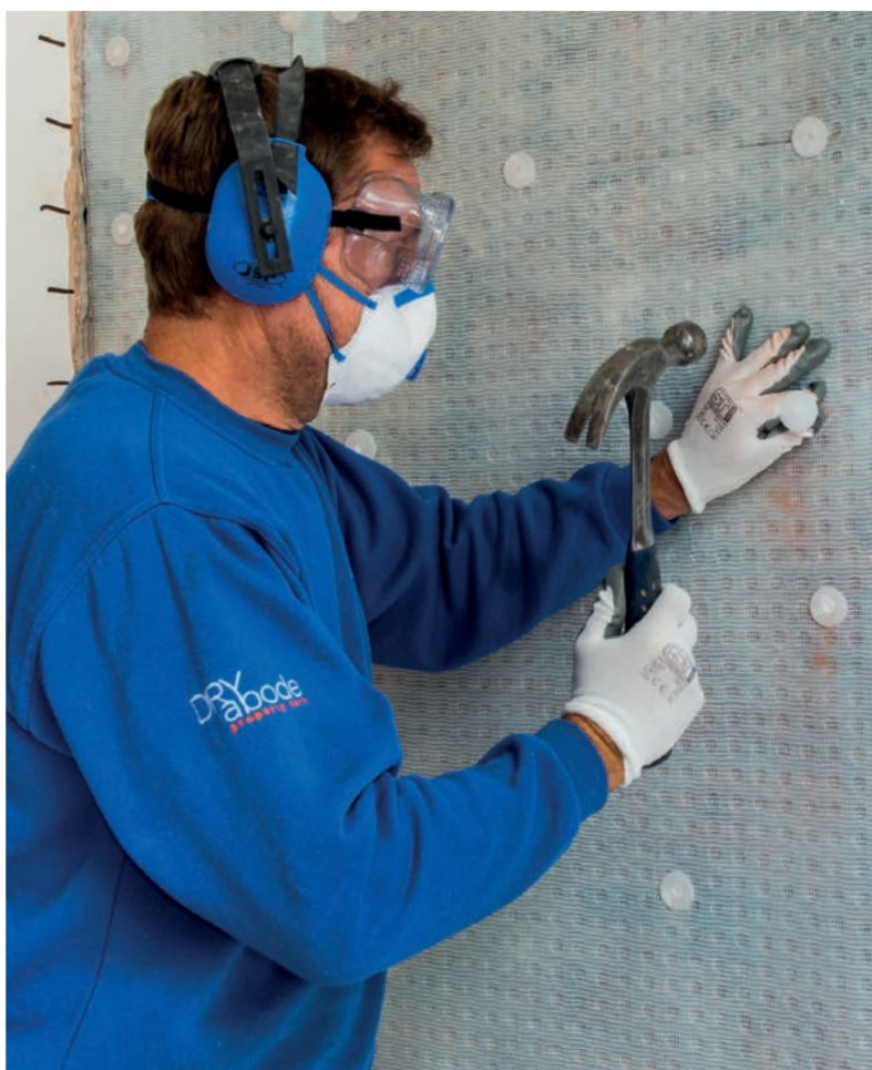
ECO Mesh Membrane being used in a damp proofing situation.
