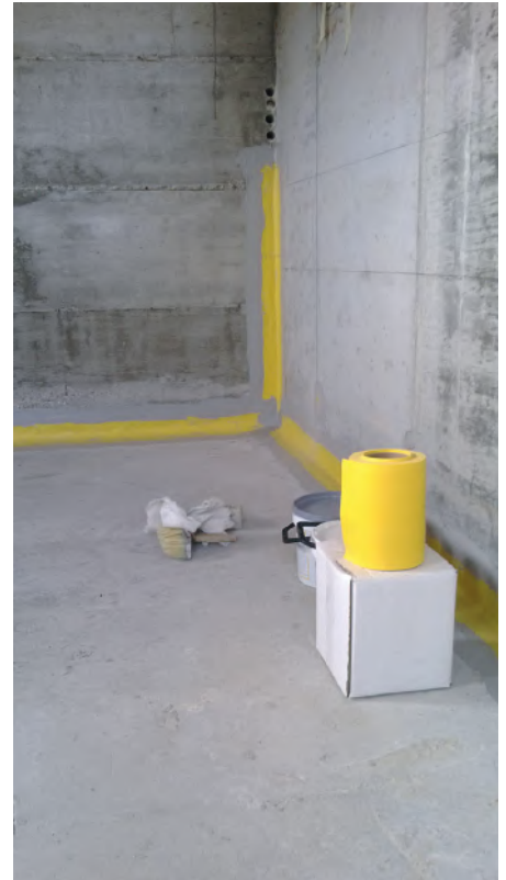
CONSTRUCTION JOINT
