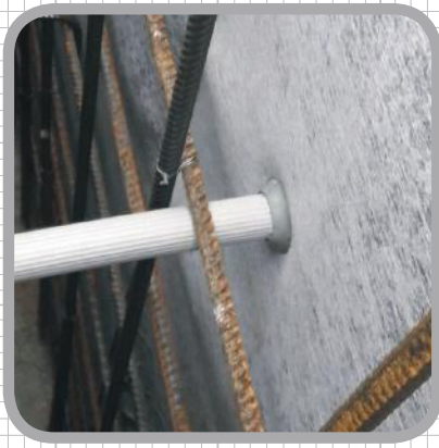
WATERPROOFING PASSING ELEMENTS
