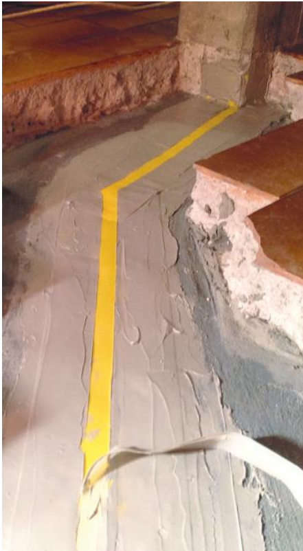
STRUCTURAL JOINT
