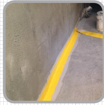
REMEDIAL TANKING OF EXISTING STRUCTURES
