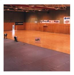
Where new floor slabs are to be laid, the use of **Wykamol Slimline** can allow the fast-track installation of floor finishes while the floor slab is still "drying down," allowing faster completion of projects.
