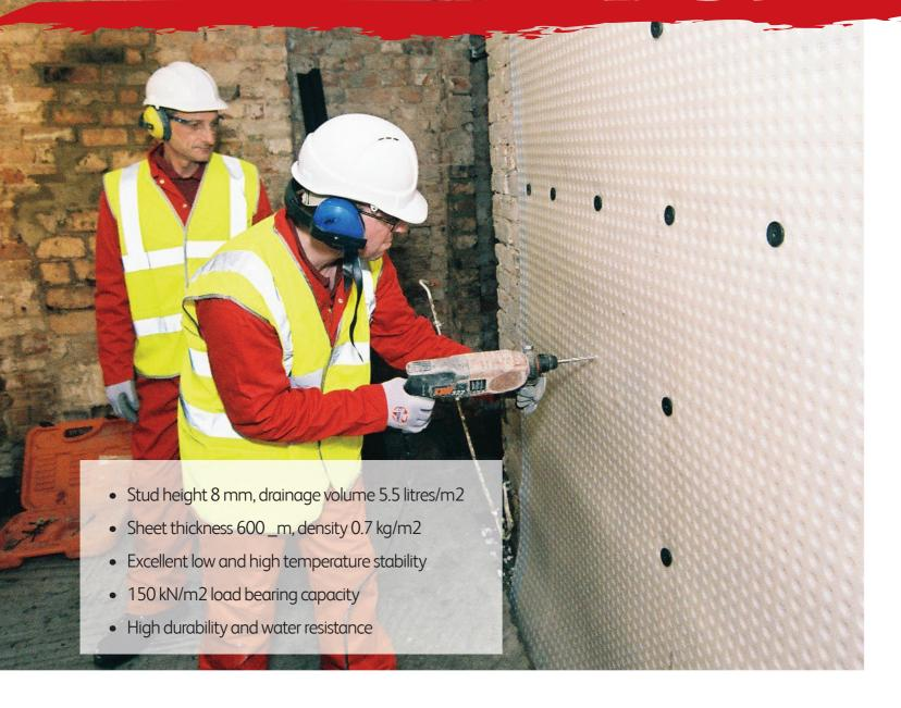
**Kontract Mesh** is a high density polyethylene membrane incorporating 8 mm studs which allows the isolation of wet walls above and below ground.
